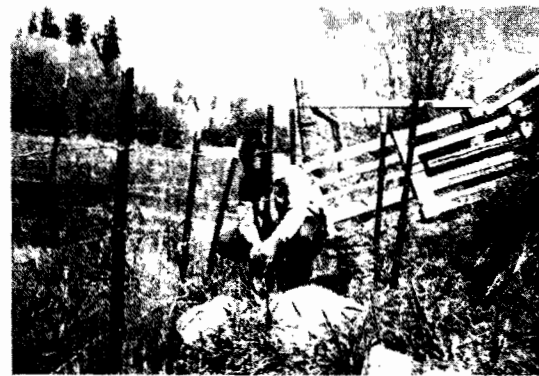
Warden Captain Lee Anderson building pedestrian bypass
