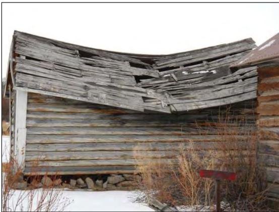
Figure 19: Collapsing roof is a safety issue
