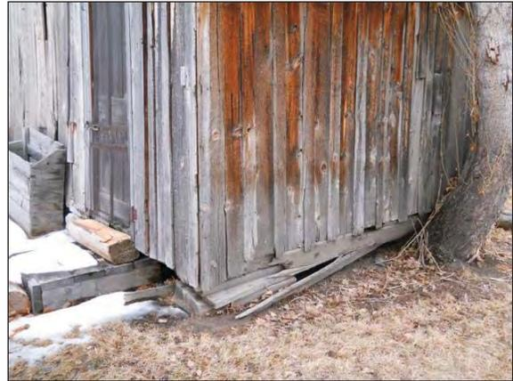
Figure 24: Iron Rod Cabin needs a foundation and weatherproofing
