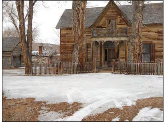
Figure 14: Poor drainage creates a sheet of ice in front of the Sedman House, an impressive structure that needs to be treated by painting
