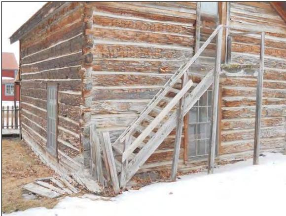
Figure 15: Rotting boards require consolidant
