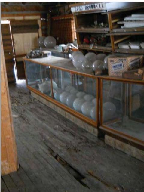
Figure 21: Charlie Bovey Building in desperate need of stabilization- floor is sunken in, endangering collections
