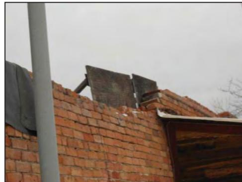
Rubber sheeting and plywood buttresses are employed to keep the brick parapet from collapsing all-together. These are temporary measures until the problem can be addressed with masonry.
