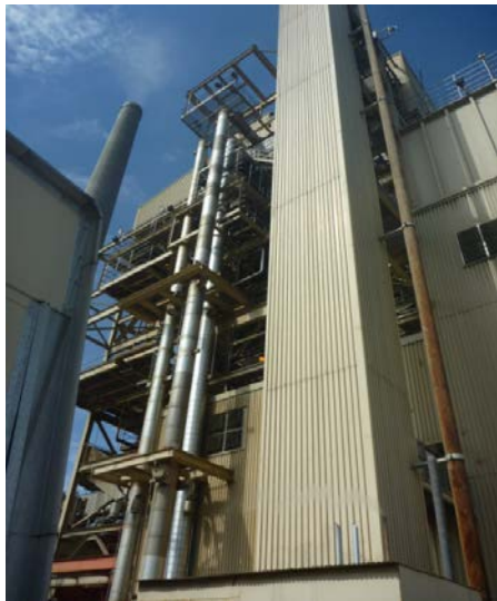
Figure 9: A look at the Corette Plant.
