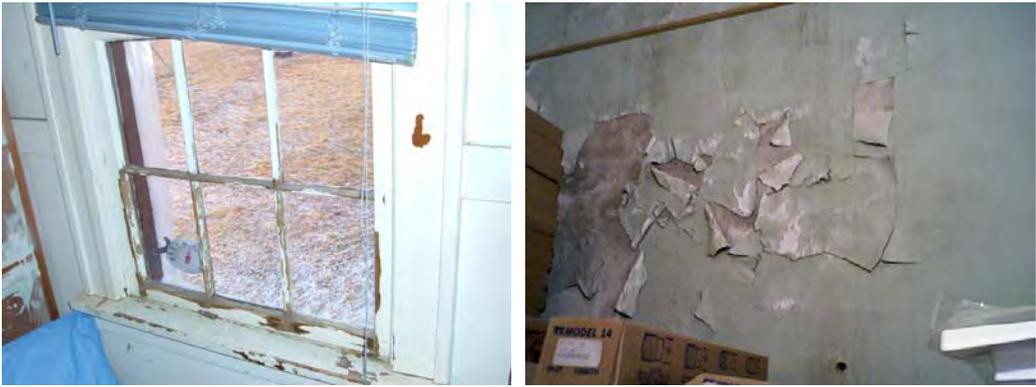
Left: Windows with failing wood frames and sashes. Right: Interior wall finish damage due to moisture penetration from the building exterior.
