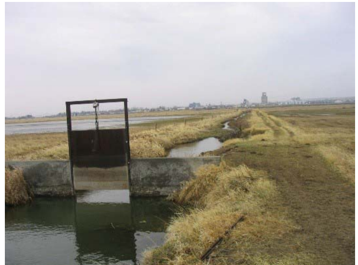
Irrigation Headgate, Near Choteau, Montana Source:WGM Group, Inc.
