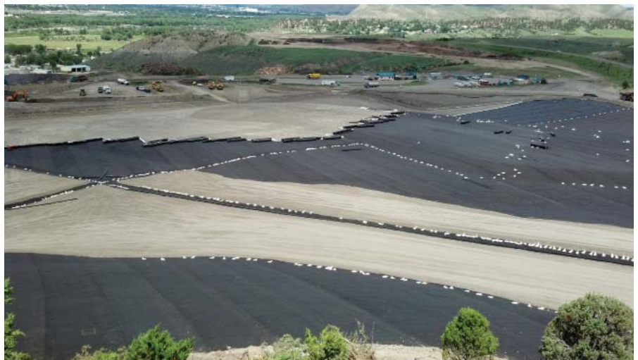
Billings Regional Landfill Phase 5 Cell
