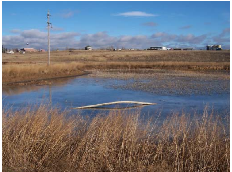
Westby, Montana Wastewater Lagoon
