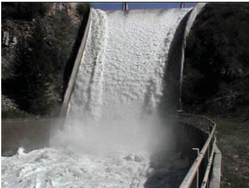
Painted Rocks Dam, near Darby, Montana
