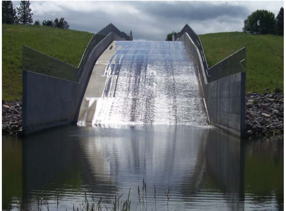
Nevada Creek Reservoir Spillway, Blackfoot River Basin, near Lincoln, Montana
