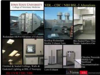
ISU-VDL BSL-3 Lab with Bio-safety Cabinets, Pass-Thru, Shower-Out & Sterilize-Out with Fail-Safe MEP/T Bldg. Systems
