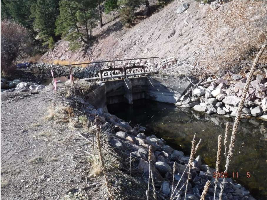
Allendale Canal Intake Structure on Flint Creek November 2020)
