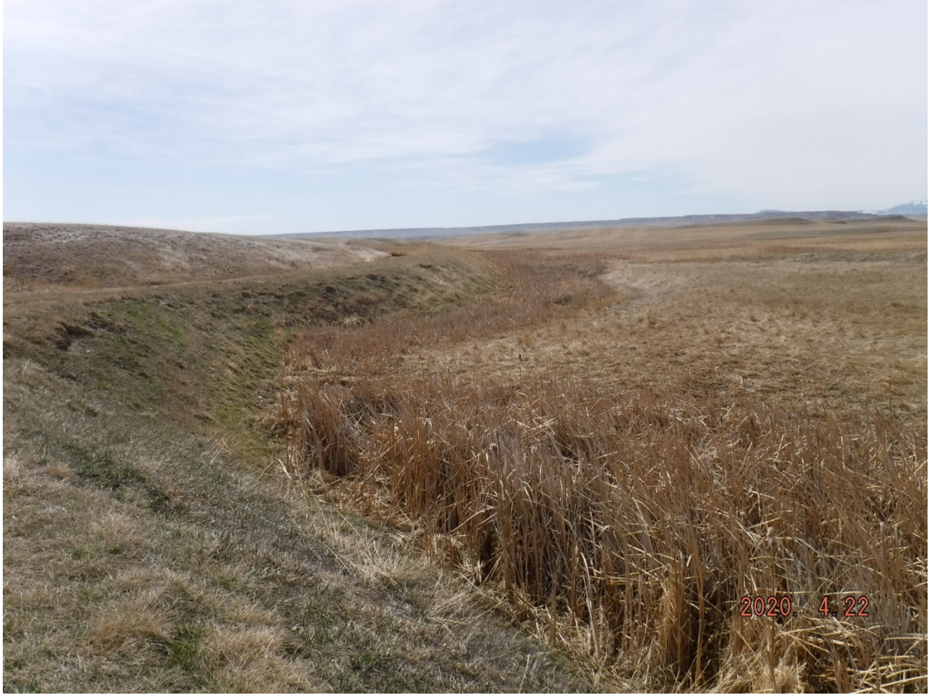
Upper Musselshell Two Dot Canal Rehabilitation (near Mexican John drainage)
