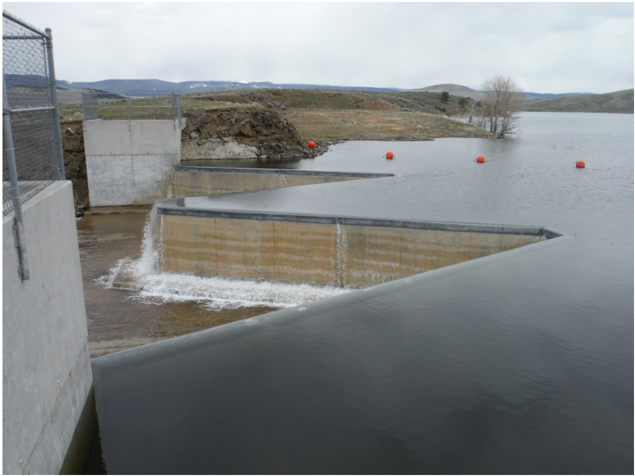
North Fork Smith River Dam, Meagher County
