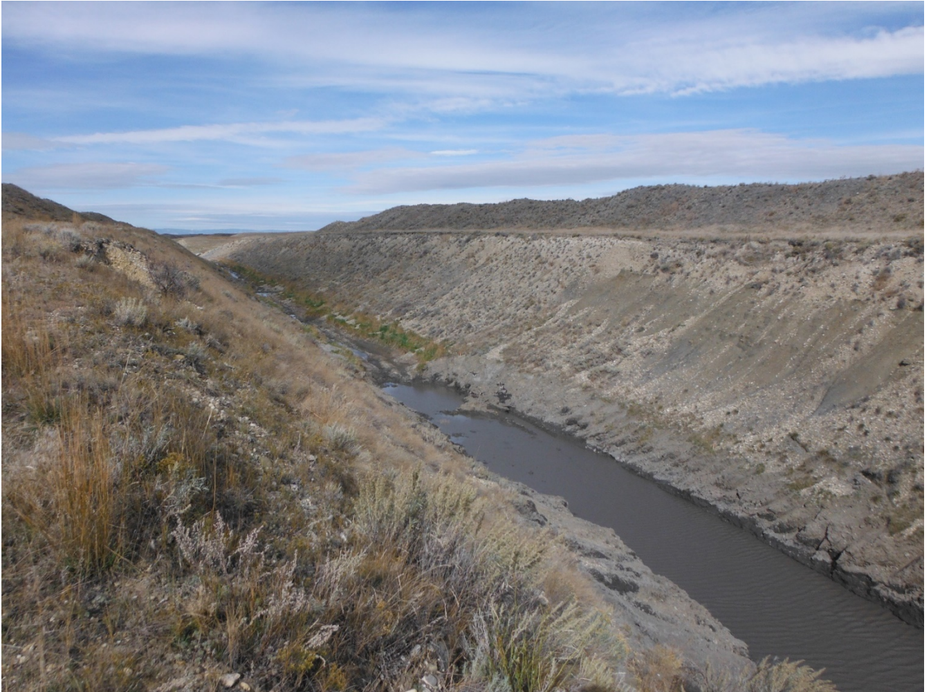
Deadman's Basin Supply Canal Rehabilitation (Phase 1 Repairs)
