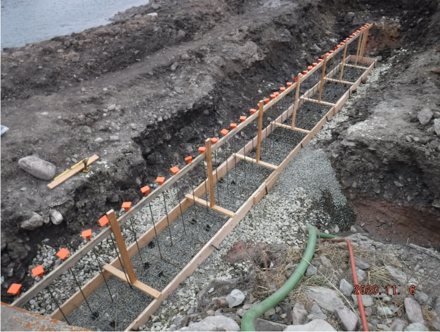
Douglas Canal Rehabilitation Construction Photos (November 2020)
