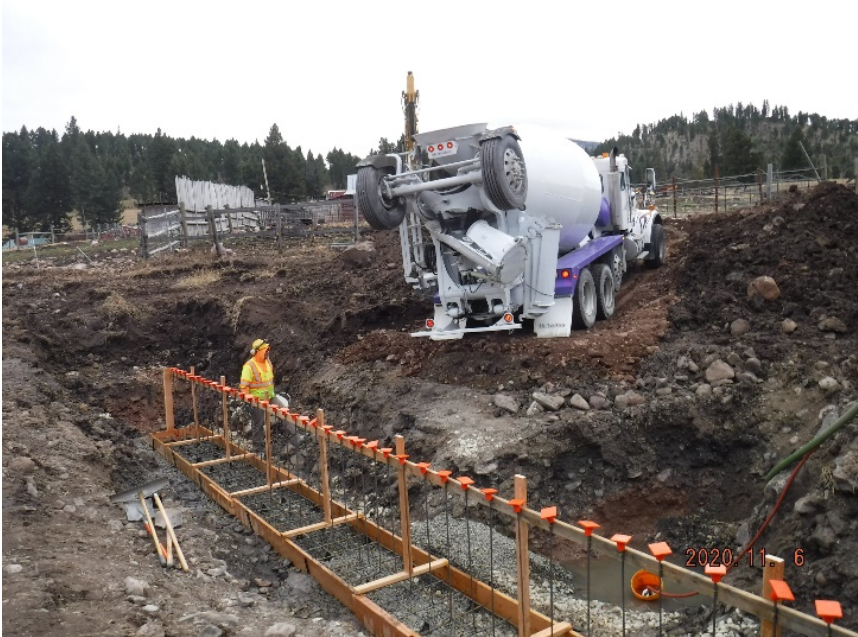
Douglas Canal Rehabilitation Construction Photos (November 2020)
