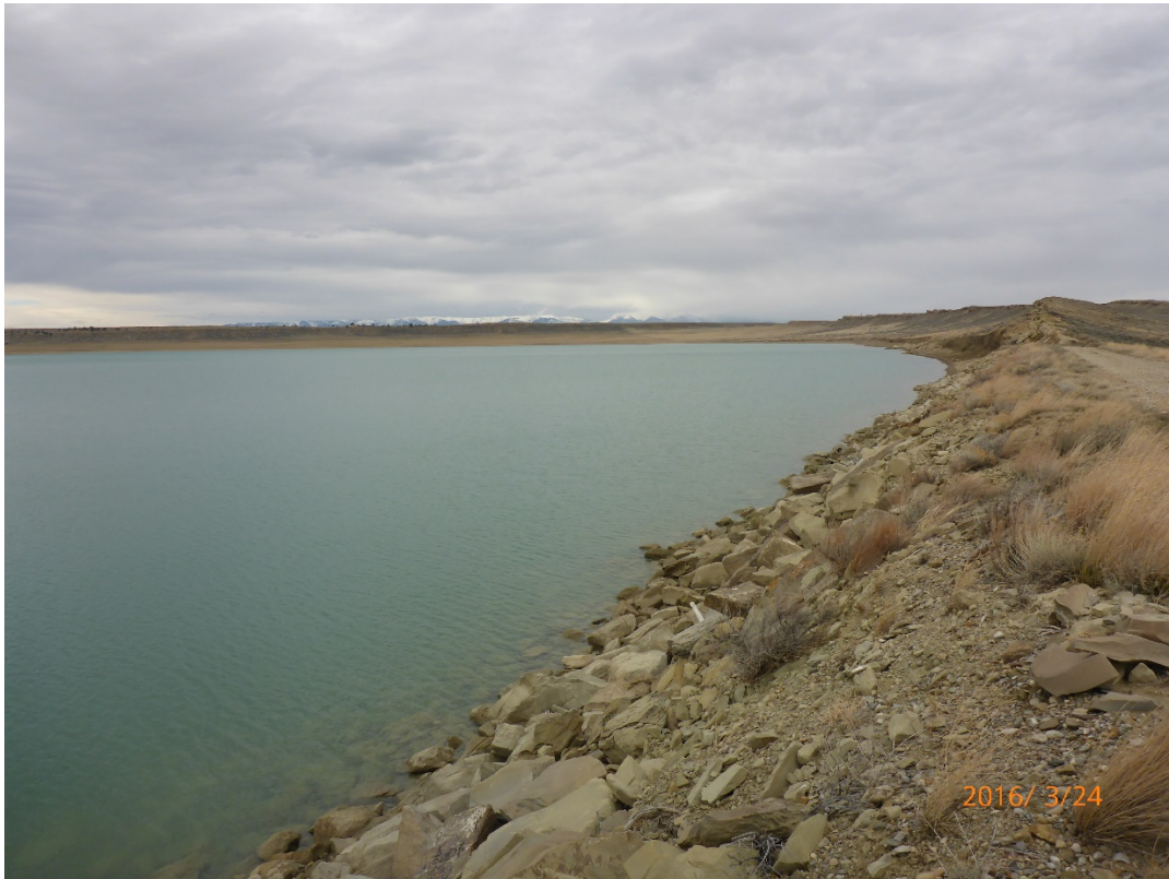
Deadman's Basin Dam (Wheatland County)
