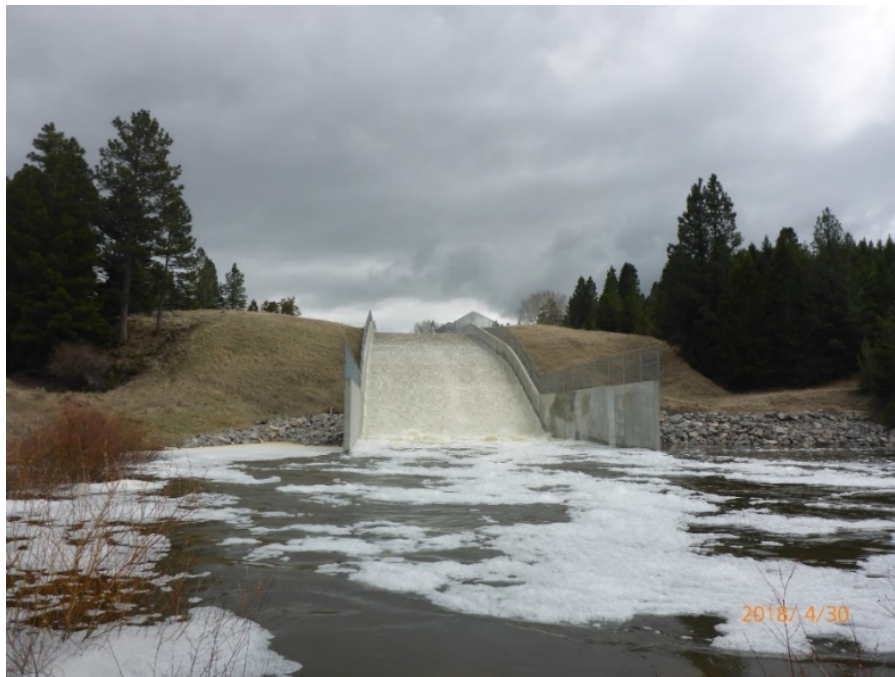
Nevada Creek Dam Spillway (Powell County)
