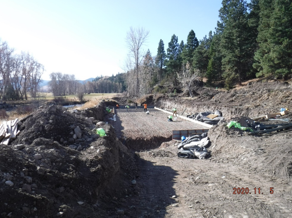
Allendale Canal Fish Screen Installation
