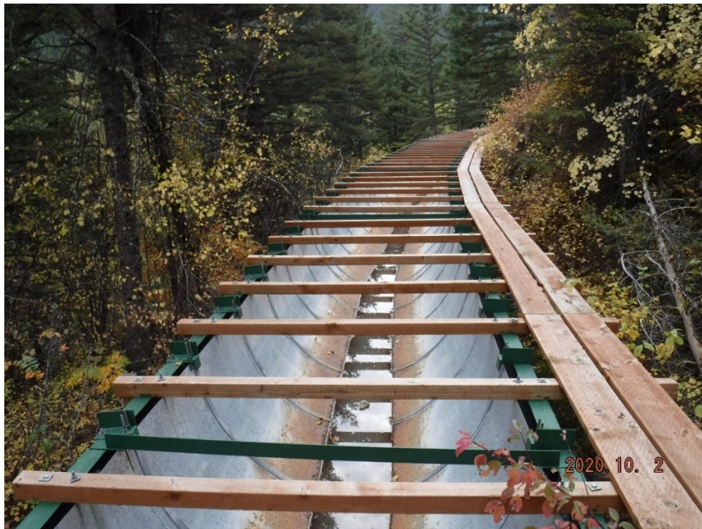
Middle Creek Cottonwood Canal North Flume (Gallatin County)
