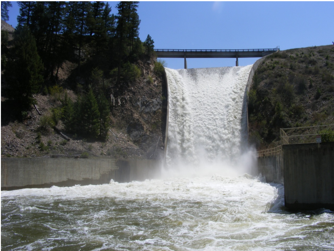
Painted Rocks Dam Spillway
