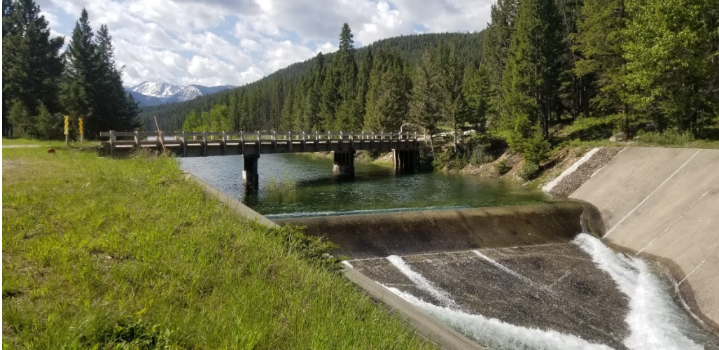
East Fork of Rock Creek Dam Spillway
