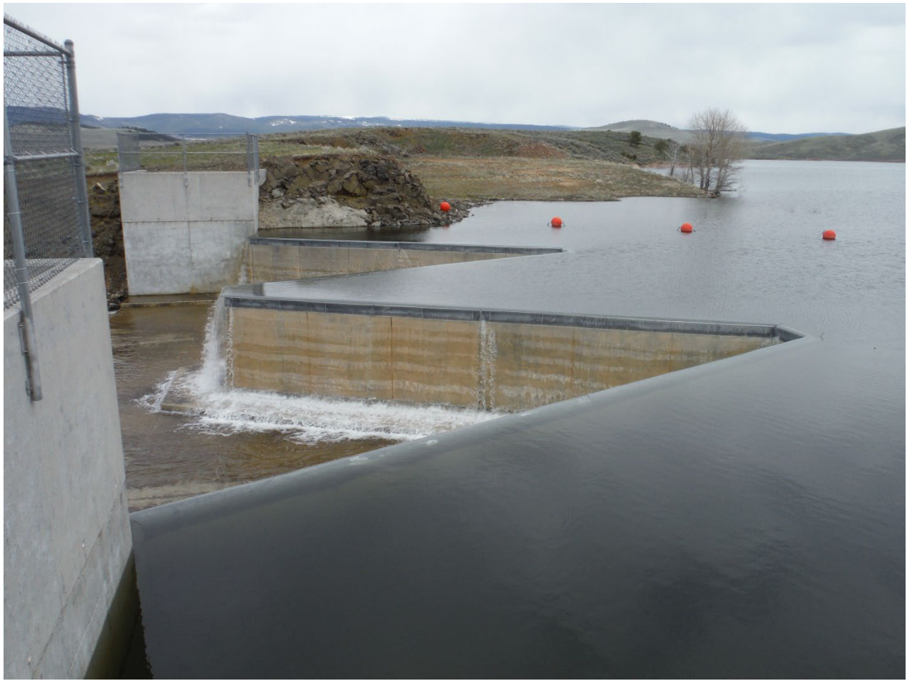
North Fork Smith River Dam, Meagher County
