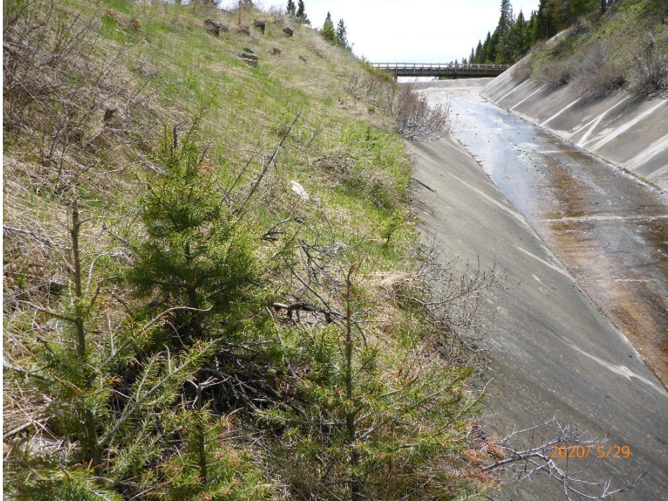
East Fork of Rock Creek Dam Spillway (Granite County)
