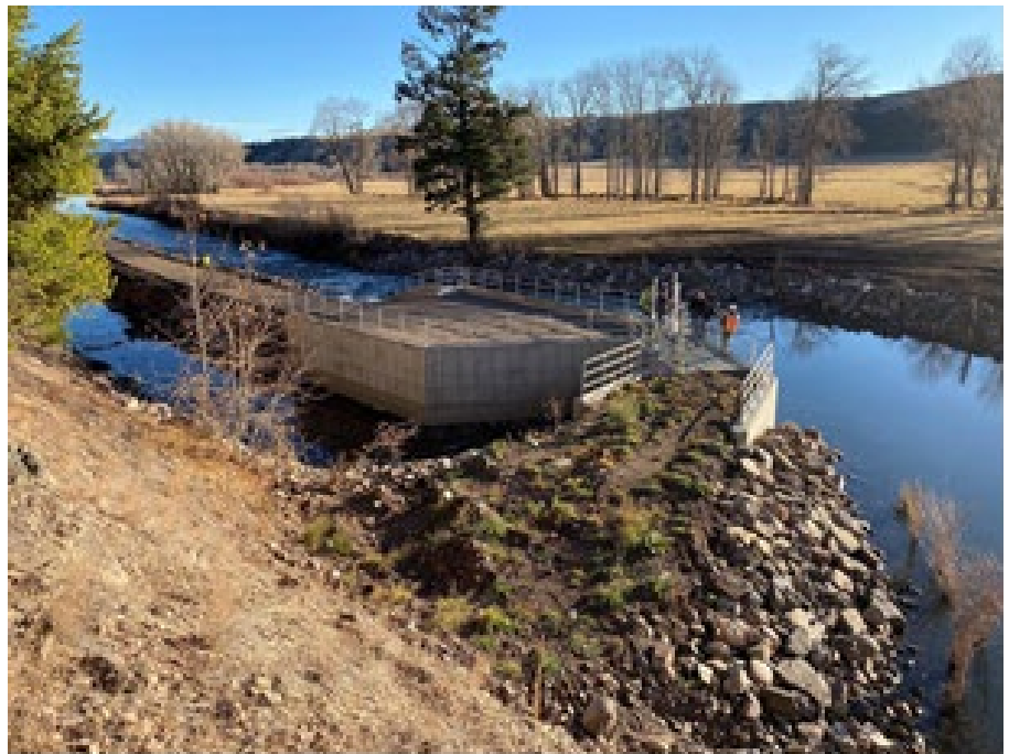
Allendale Canal Intake Structure on Flint Creek
