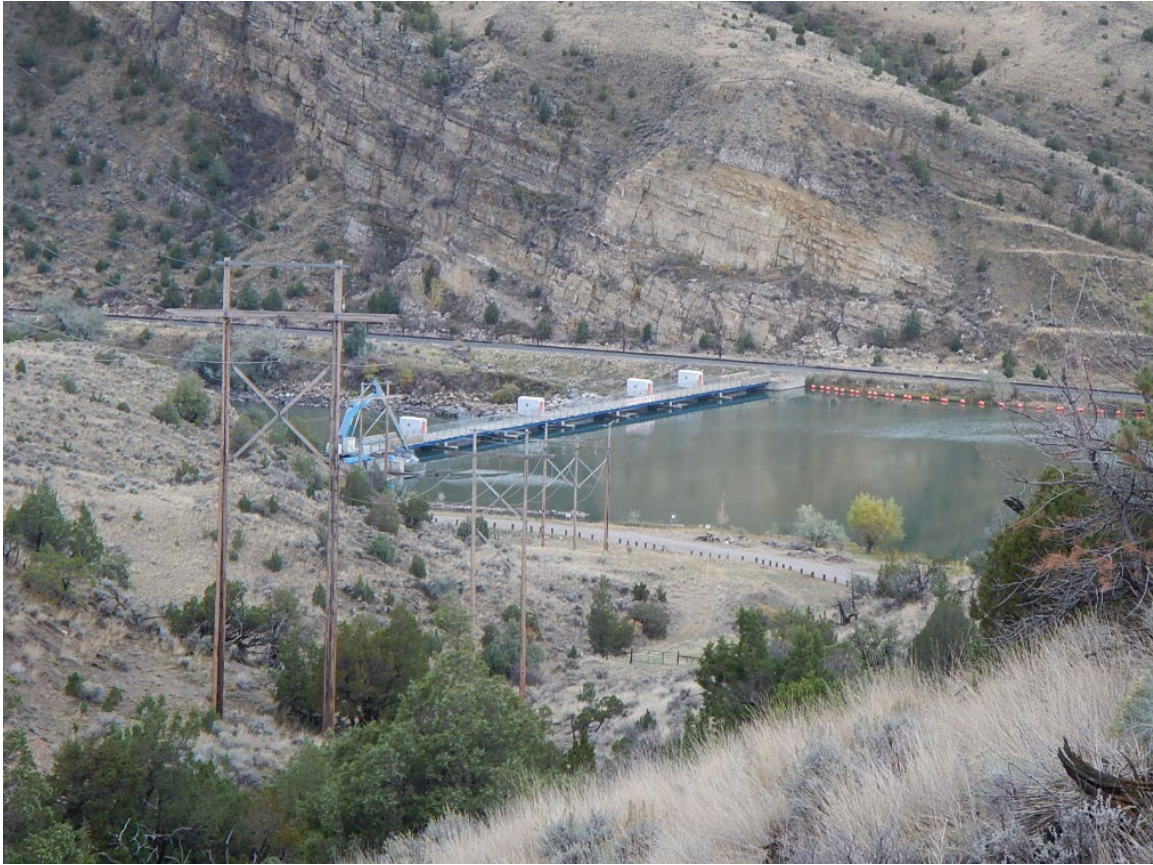
Broadwater Power Project, Missouri River near Toston, Montana
