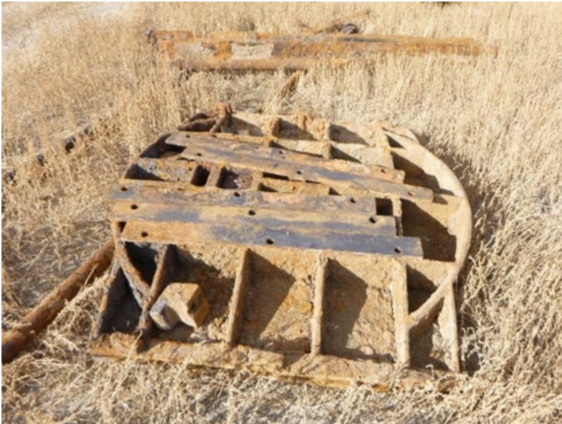
Frenchman Dam. 60-year-old Operating Gate, Recently Replaced
