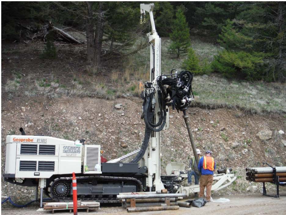
Geotechnical Investigation Drilling at East Fork of Rock Creek Dam (Granite County)
