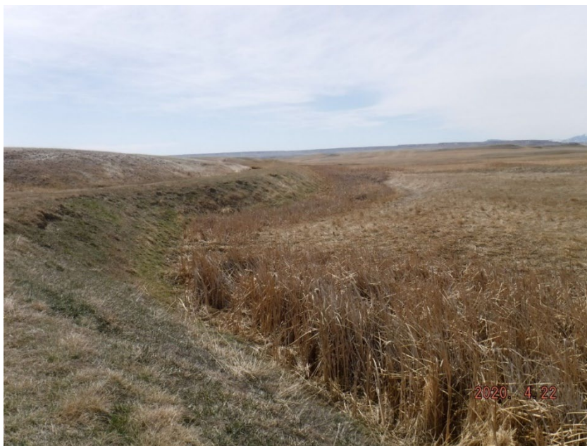
Upper Musselshell Two Dot Canal (near Mexican John drainage)
