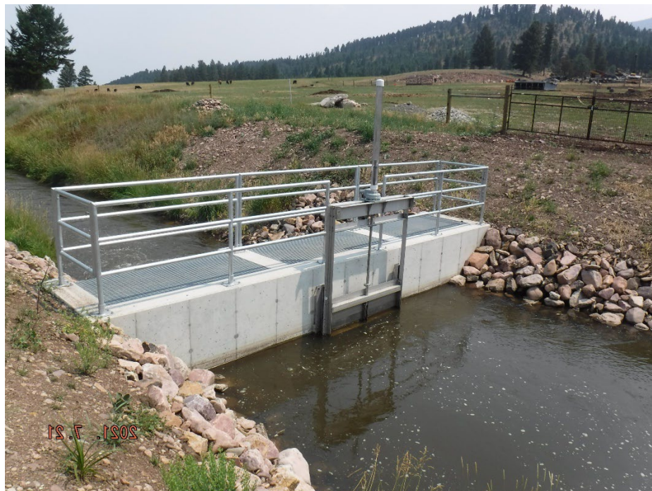
Nevada Creek Douglas Canal - New Intake Structure
