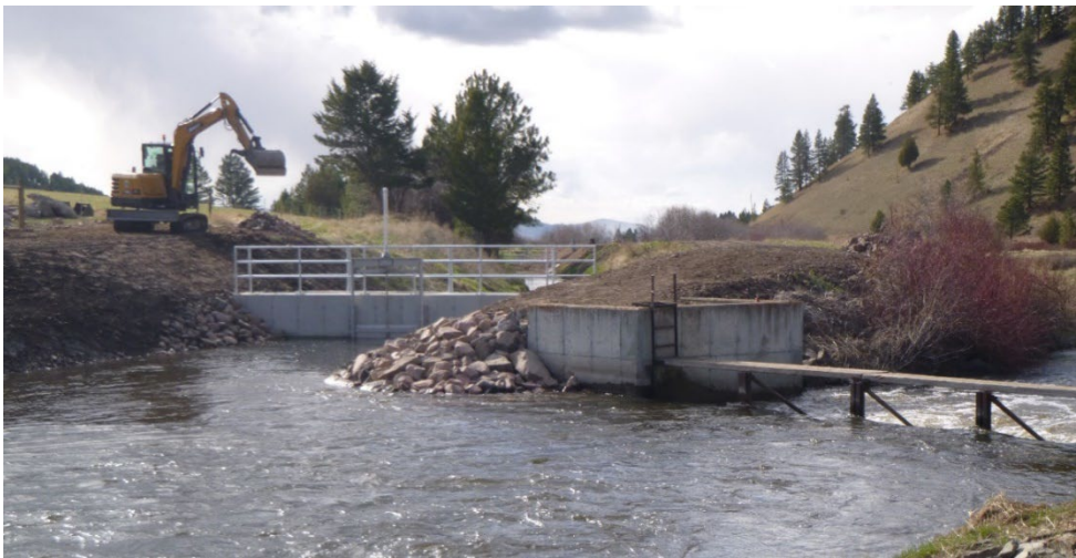
2021 Douglas Canal Rehabilitation, Nevada Creek State Water Project (Powell County)
