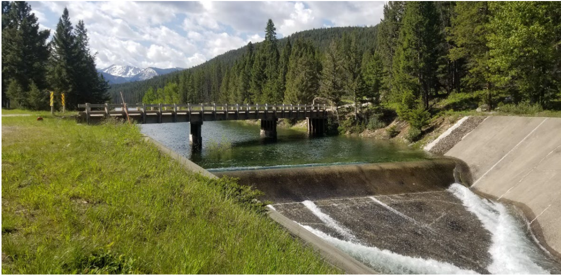
East Fork of Rock Creek Dam Spillway
