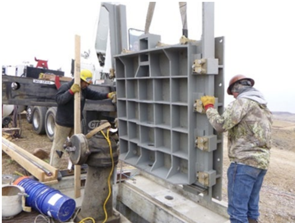
Frenchman Dam. Workers installing new operating gate.
