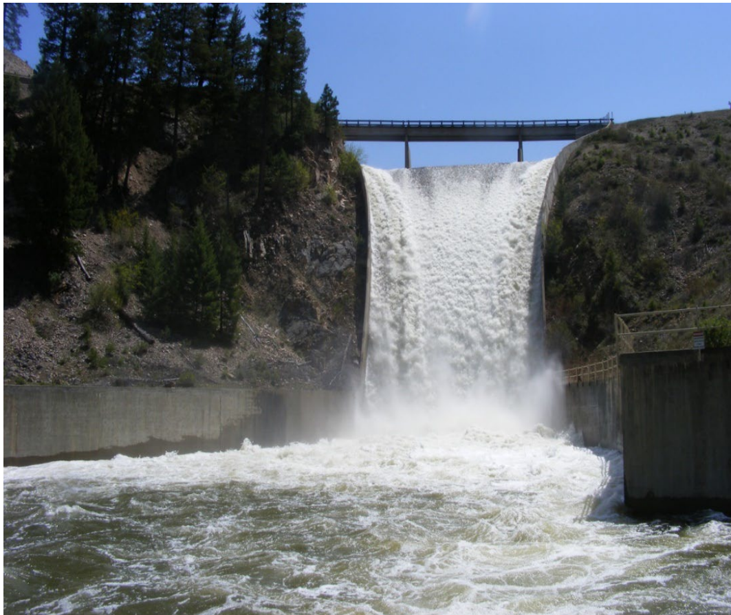
Painted Rocks Dam Spillway
