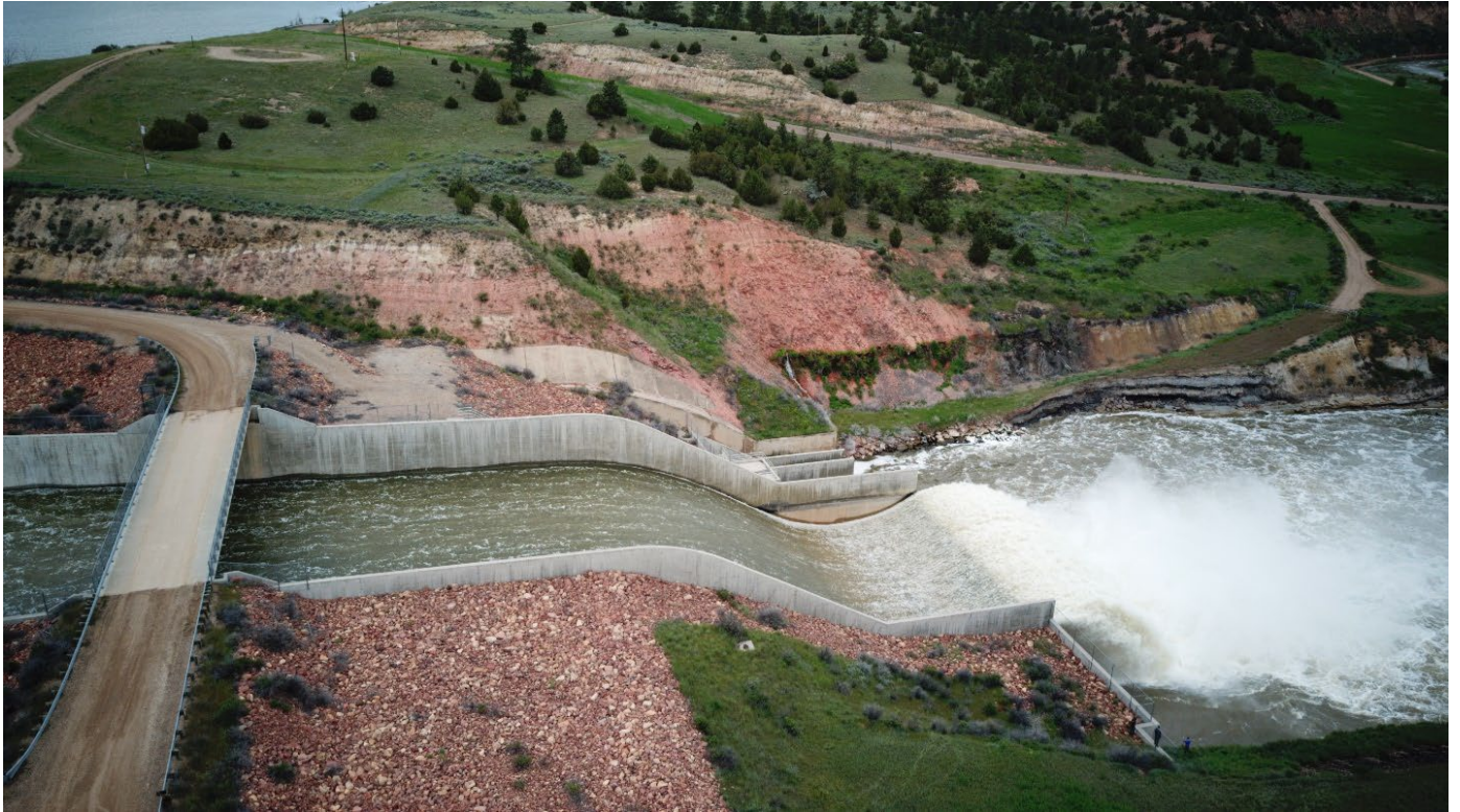
Aerial view of Tongue River Dam Spillway
