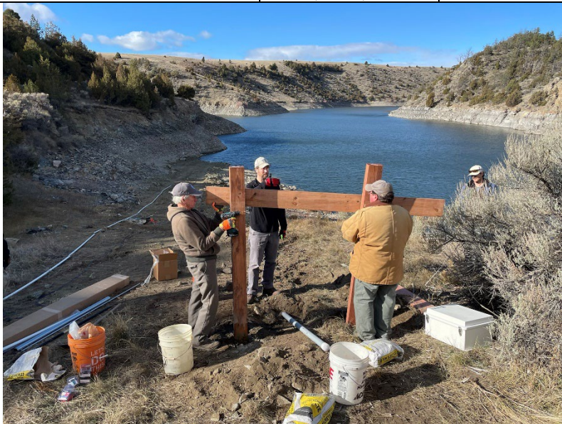
Willow Creek Dam – Installing Reservoir Transducer in 2021
