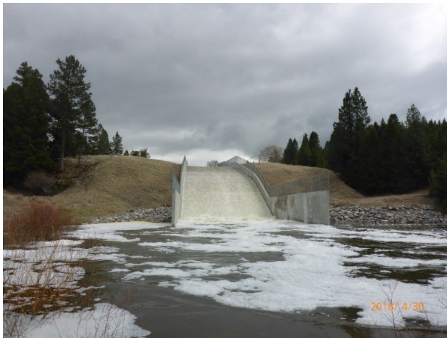
Nevada Creek Dam Spillway (Powell County)
