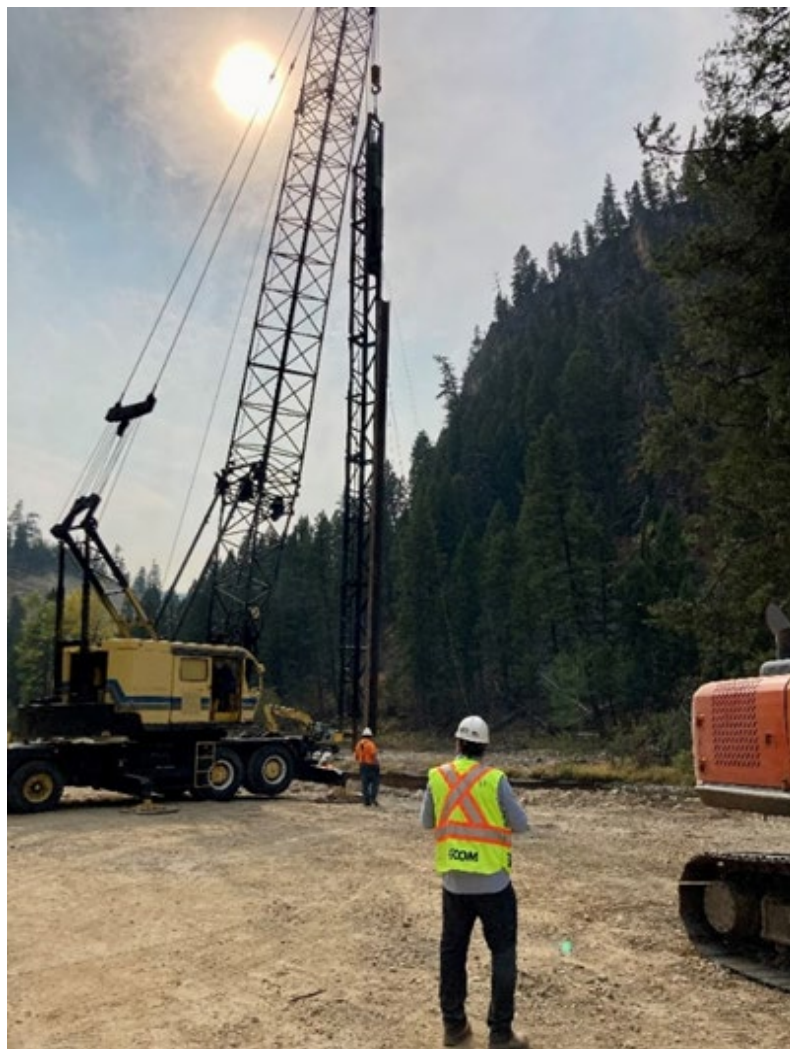
Painted Rocks Dam-Driving Piling for New Bridge Abutments for Improved Access.
