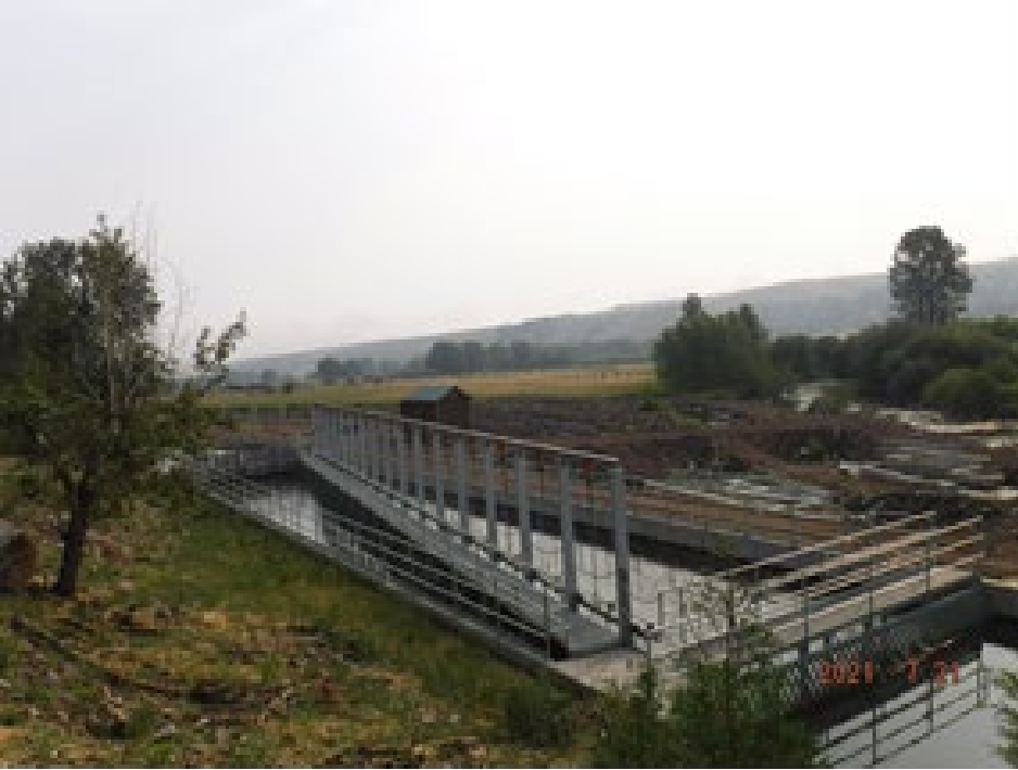
Allendale Canal Fish Screen Installation
