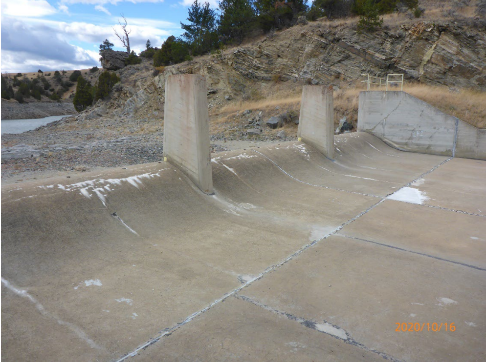
Willow Creek Dam – Upper Portion of Spillway
