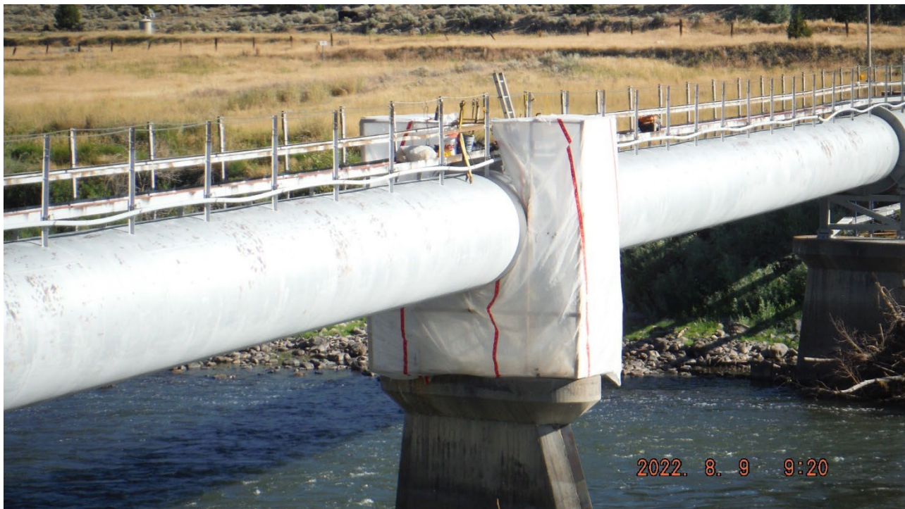
Broadwater-Missouri Project- Repair and Maintenance on Missouri River Pipe Span
