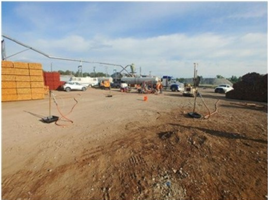
Chemical oxidation injection work as part of groundwater remedy implementation at the KRY Site
