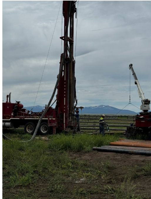
Drilling exploratory wells for ASR.
