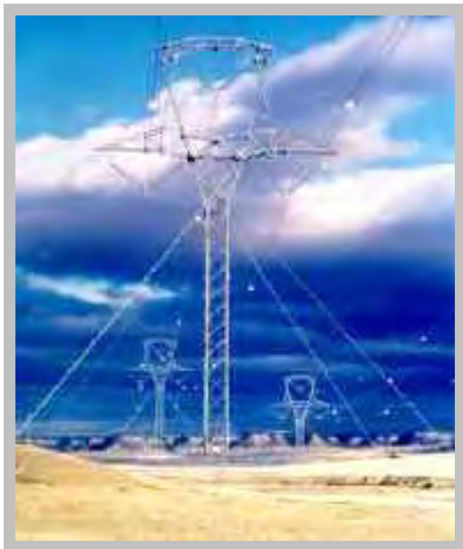
Montana transmission lines. Photo courtesy of Tom Ring, DEQ.
