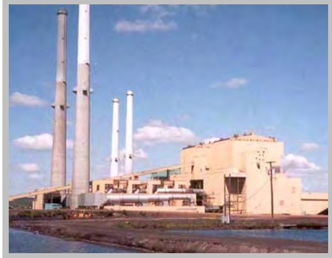
Colstrip plant in Eastern Montana. Photo courtesy of the DEQ.
