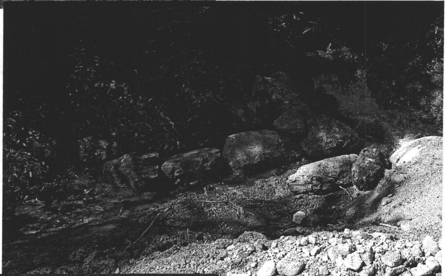
Rap rip is used to stabilize soils at culvert inlets and outlets.
