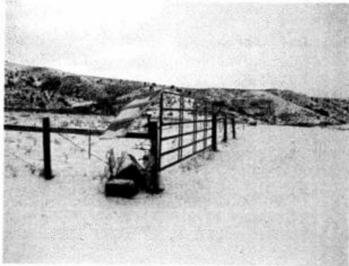
Figure 1. Photos of a five wire high tensile electric fence that has proven effective for managing bison in grazing pasture situations. The fence is 48" high with an 18" bottom wire. Note the placement of solar charger and the gate is mounted higher than the fence.
