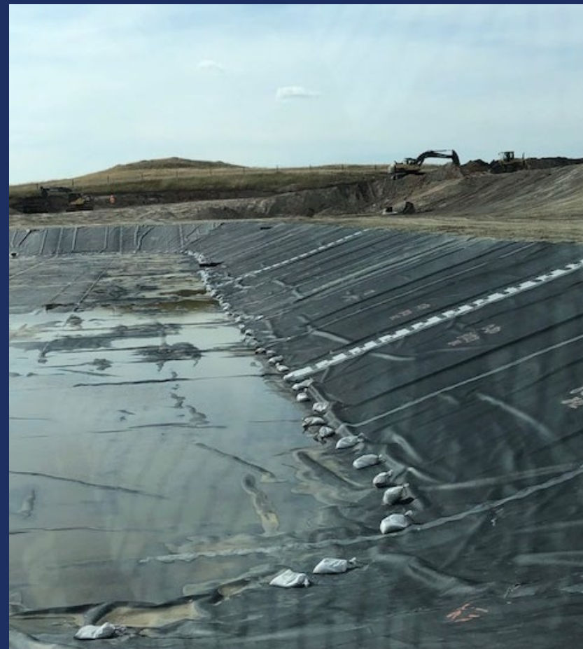
Wibaux Wastewater Lagoon. Photo credit: MCEP. 2023
