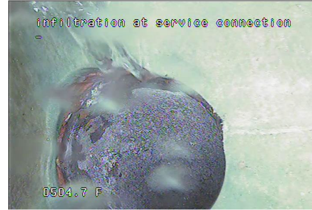
Wastewater system. Photo credit: City of Deer Lodge, 2024.
