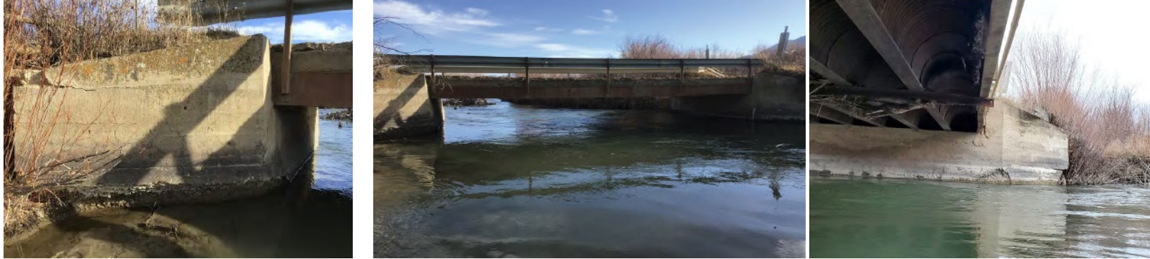
Bridge. Photo credit: Madison County, 2024.
