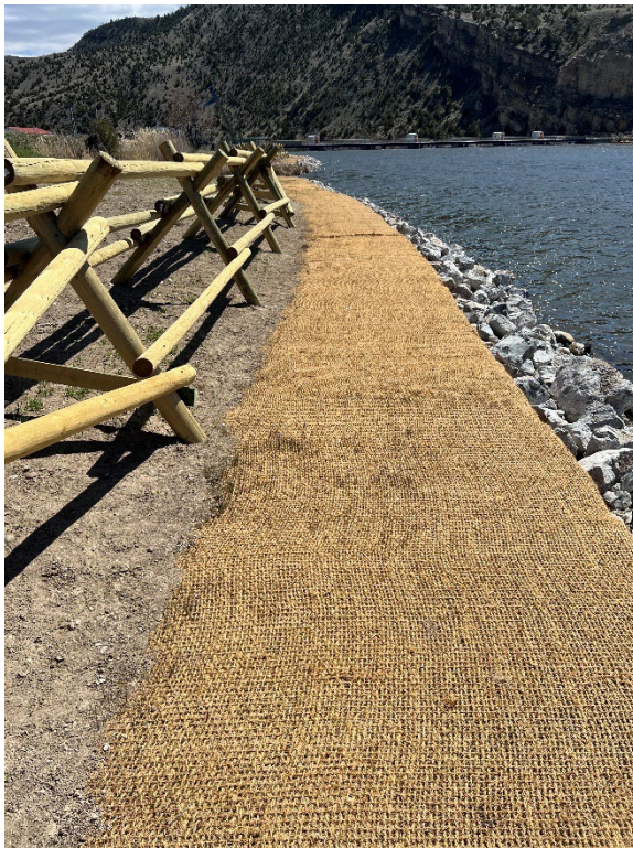
Shoreline Stabilization – BLM's Upper Toston Recreation (near Toston Dam), Broadwater County
