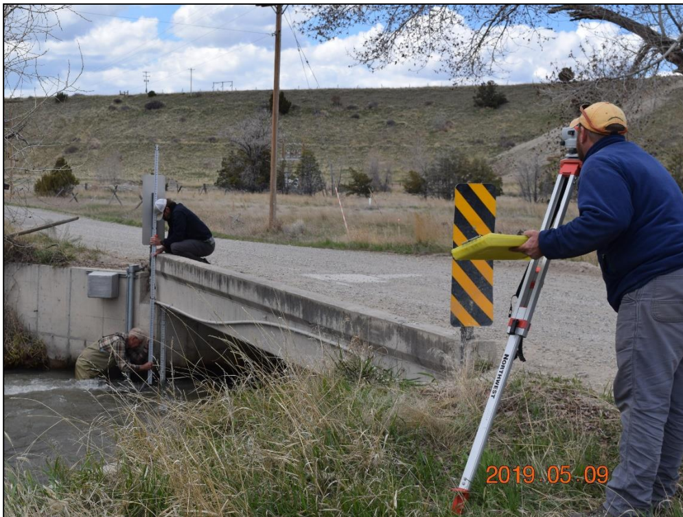
Figure 4. Gage 41I 03500 Deep Creek near Townsend during installation.
