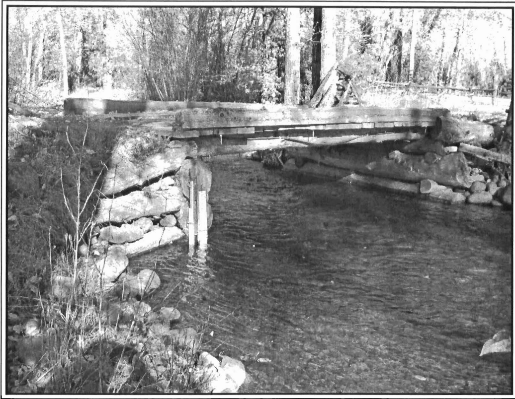
Figure 2. Kendall Bridge October 26, 2005. The Aquarod® is housed in the metal pipe attached to the left bridge abutment.
