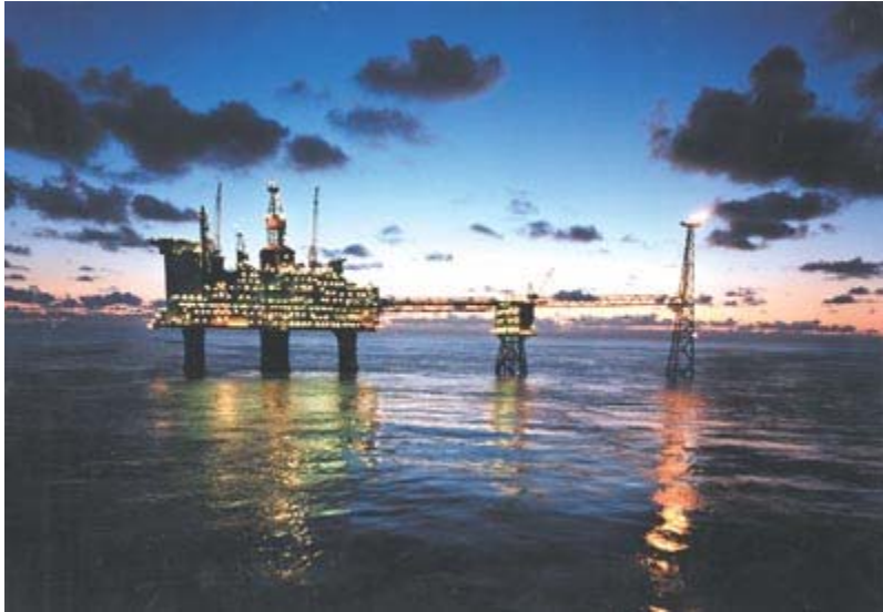
Figure 4-4. Photo of Statoil's Sleipner Project (Injecting CO 2 in a Reservoir Beneath the North Sea Since 1999).
