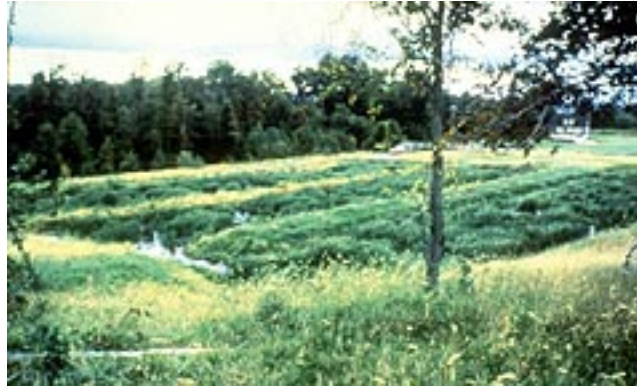
Figure 1-6. Constructed Wetland for Mine Water Discharge Treatment.
