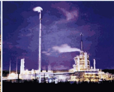
▲ Wabash River Coal Gasification Plant
