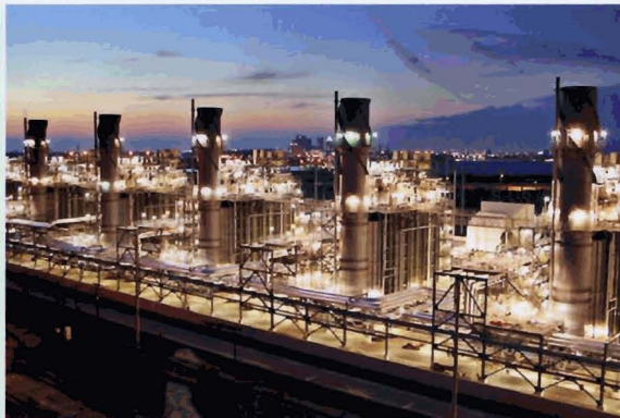
▲ Tampa Electric's Polk Power Station
