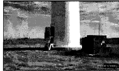
Pad Mounted Transformer at Base of Wind Turbine
